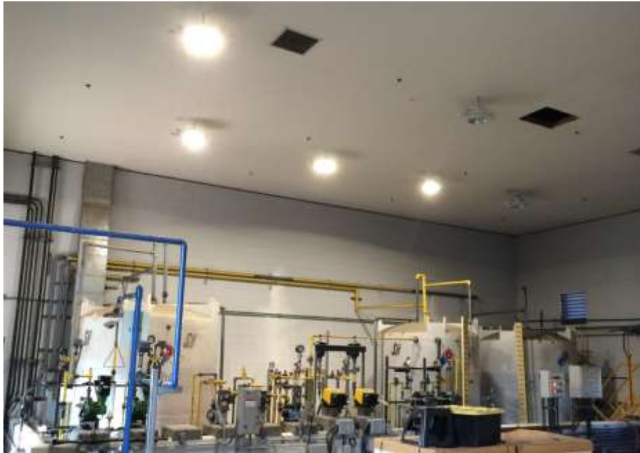
LEDs installed at RP4's chemical storage room
