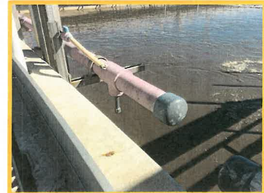
Out of Service Surface Sprayer Pipeline
