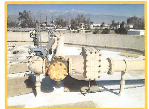
Digester No. 6 Flame Arrestor
