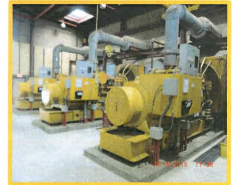
Back up Generators at RP-1
