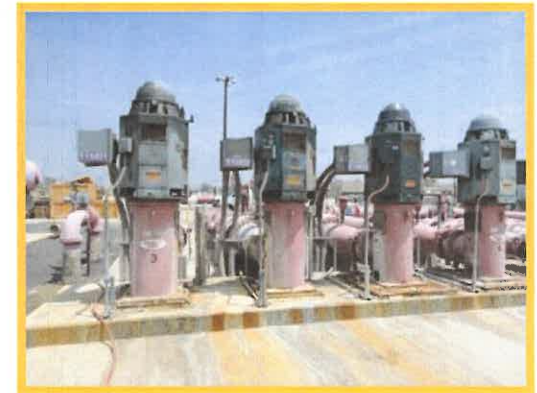
Recycled Water Pump Station Motors
