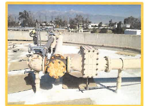
Digester No. 6 Flame Arrestor
