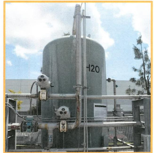
Deterioration of Surface Coating on Process Vessel
