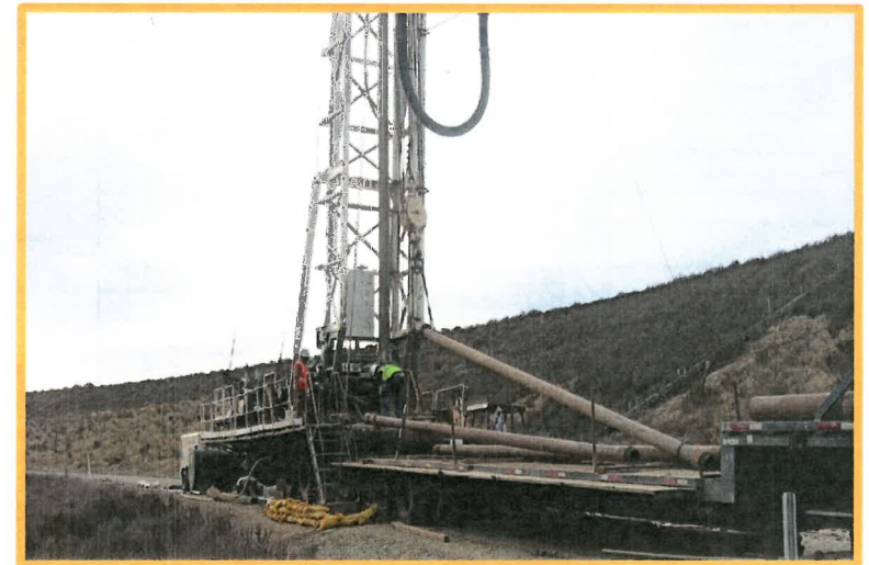
Past Construction of a Monitoring Well for San Sevaine Basin South End of Basin 5
