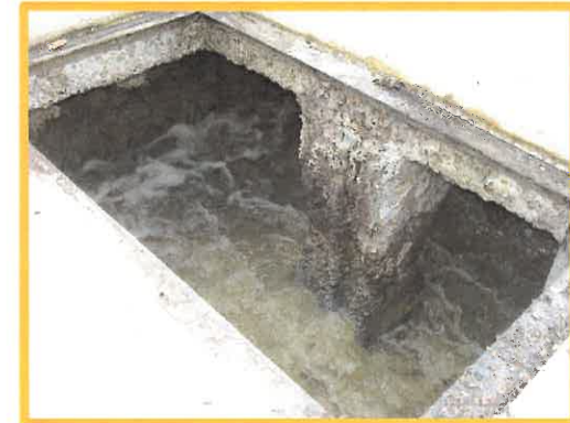
Corroded Concrete Deck
