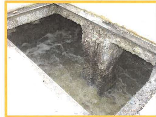
Corroded Concrete Deck
