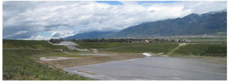
*The IEUA region is underlain by large groundwater basins that can retain rain and runoff as well as recycled water. Development limits natural recharge, but constructed recharge basins help to offset those losses.*
