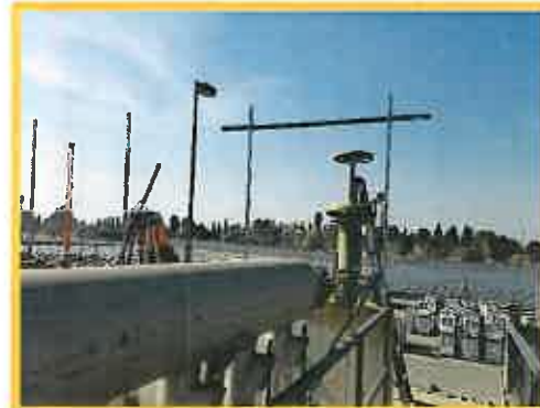
Aeration Basin New Conduit Installation
