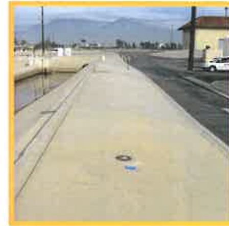
RP-1 North Access Road to be Widened
