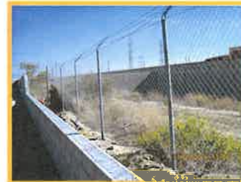
RP-4 Wall to be Completed
