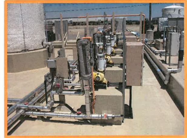
Replace Existing SHS Pumps
