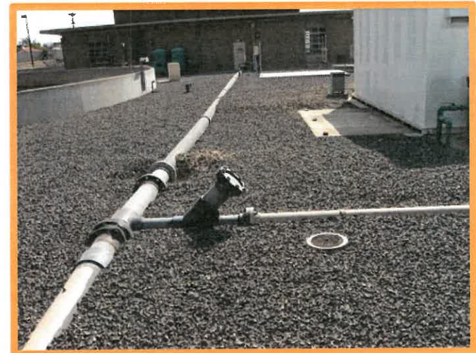
TWAS Line to be Replaced
