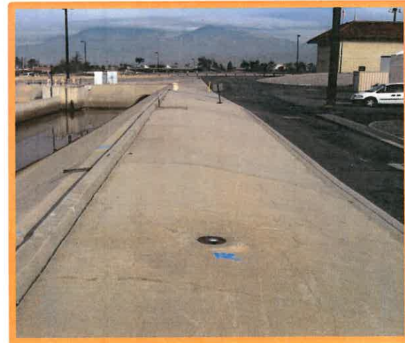
Wash Water Basin Wall to be Modified
