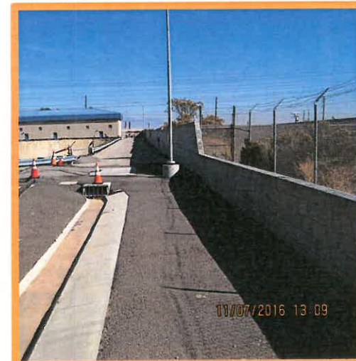
Stem Wall to be Completed to Full Height
