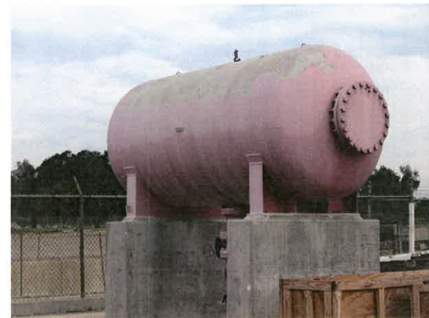
Non-operational surge tank
