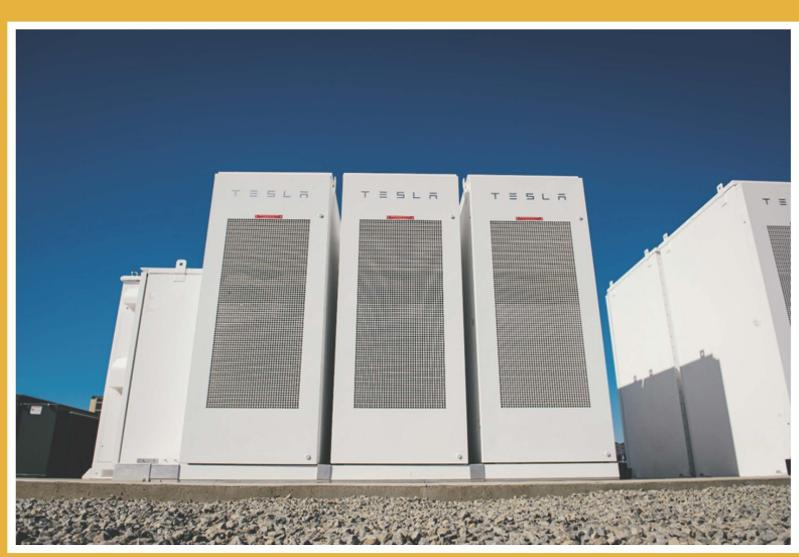
Construction of the RP-5 battery storage project was completed in June 2016. Storing electricity during periods of low grid demand and supplementing RP-5's power needs during peak periods saved IEUA approximately \$17,000 in the last half of 2016.
