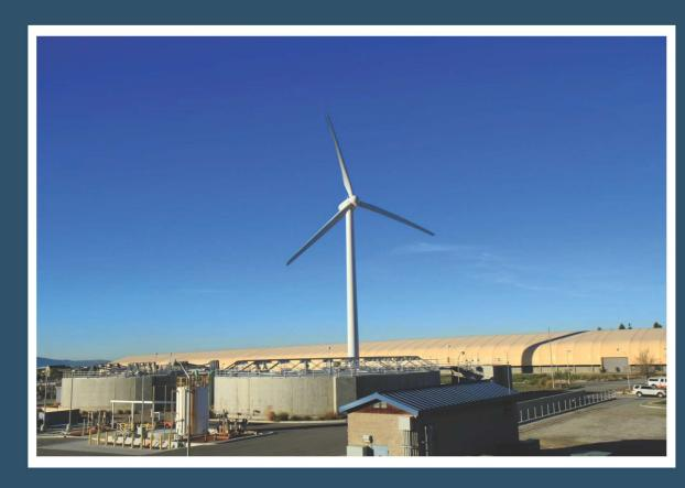
IEUA's Regional Water Recycling Plant Number 4 (RP-4) is located adjacent to IERCF in Rancho Cucamonga, California. The facility houses a 1 MW wind turbine to provide renewable power to the facility. A 2.5 MWh battery storage system is expected to complete construction at RP-4 in 2017.
