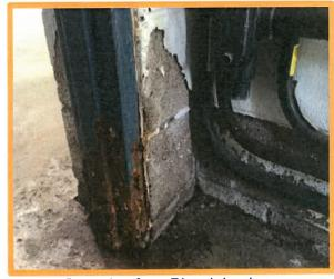
Corrosion from Bleach Leakage
