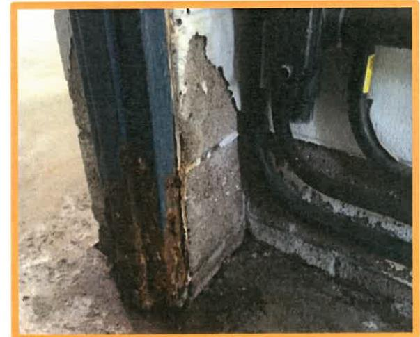
Corrosion from Bleach Leakage
