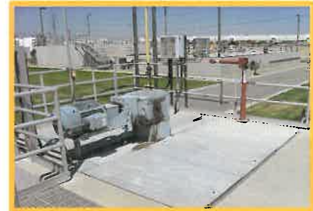
CCB INLET STRUCTURE
