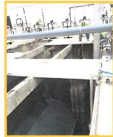
CORRODED CONCRETE
