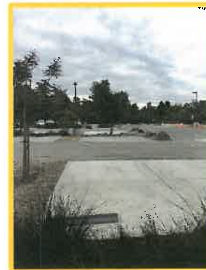
RECENTLY POURED SLABS AND REMOVED ASH TREES
