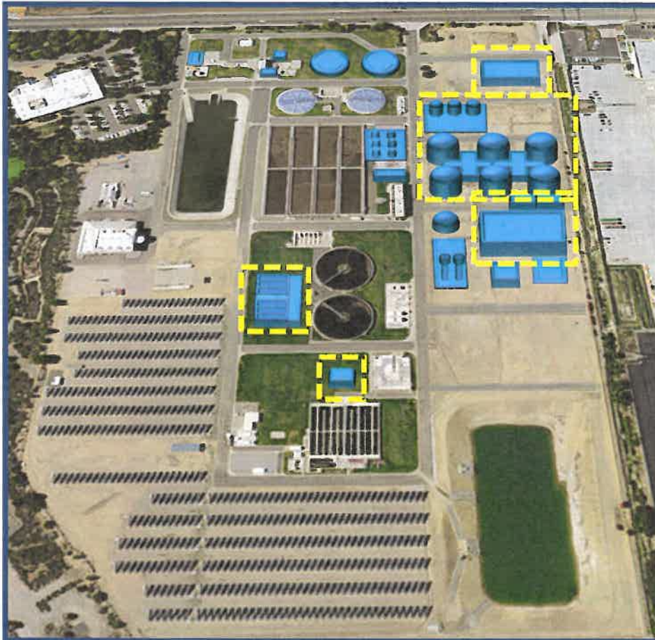
RP-5 Liquids Expansion and Solids Facility
