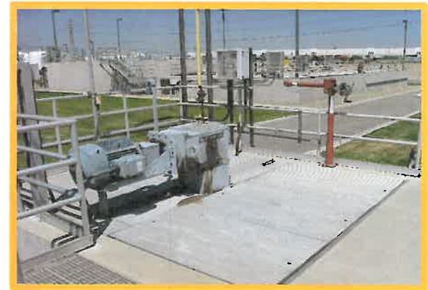
CCB INLET STRUCTURE
