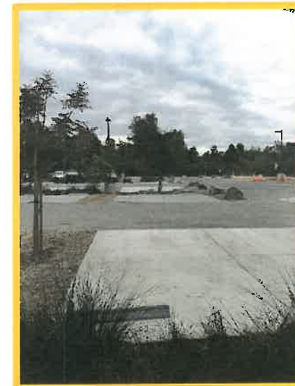
RECENTLY POURED SLABS AND REMOVED ASH TREES
