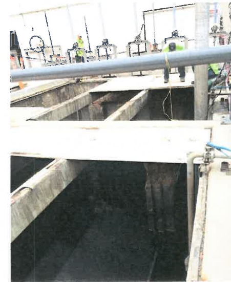
Corroded Concrete
