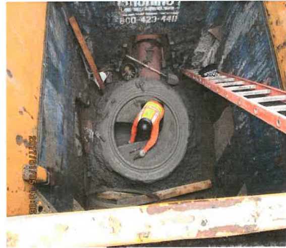
New 18-in Manhole Base
