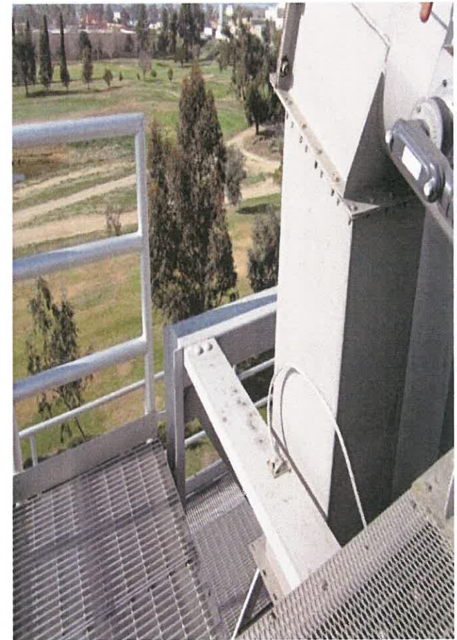
Location of Additional Railing
