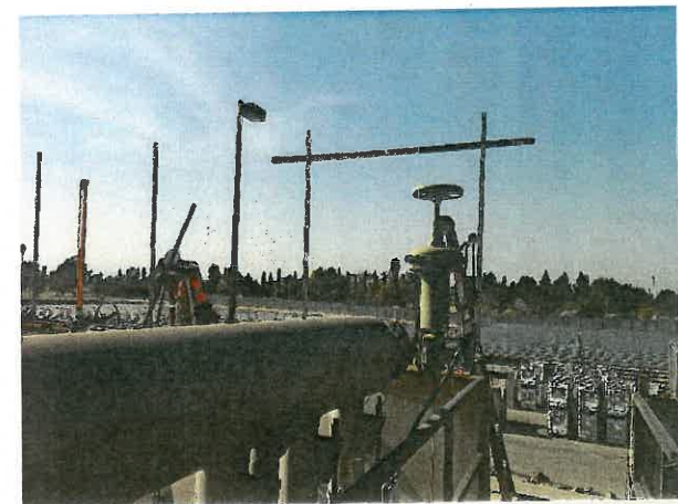
Aeration Basin New Conduit Installation
