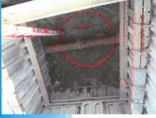
Connection Point for New 8-In Sewer Lateral
