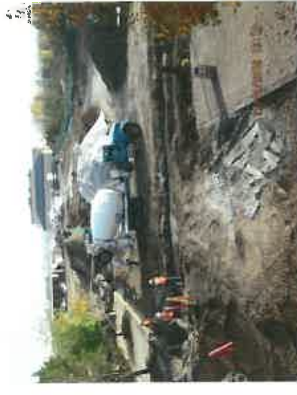
Trench Backfill and Compaction
