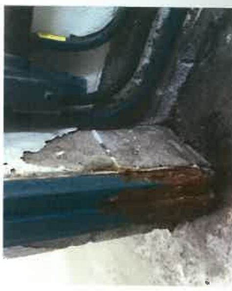
Corrosion from Bleach Leakage
