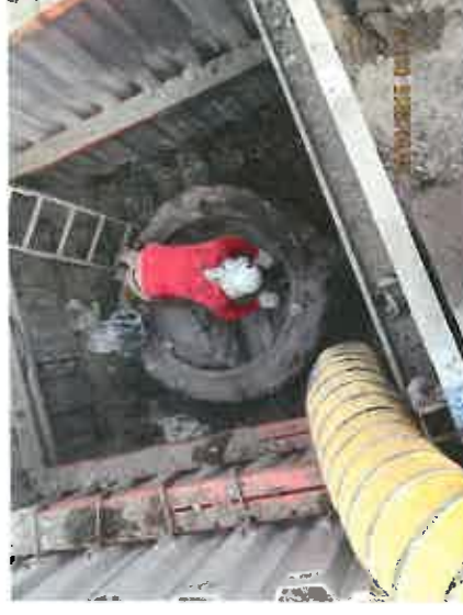
New Manhole Construction Over the Existing
