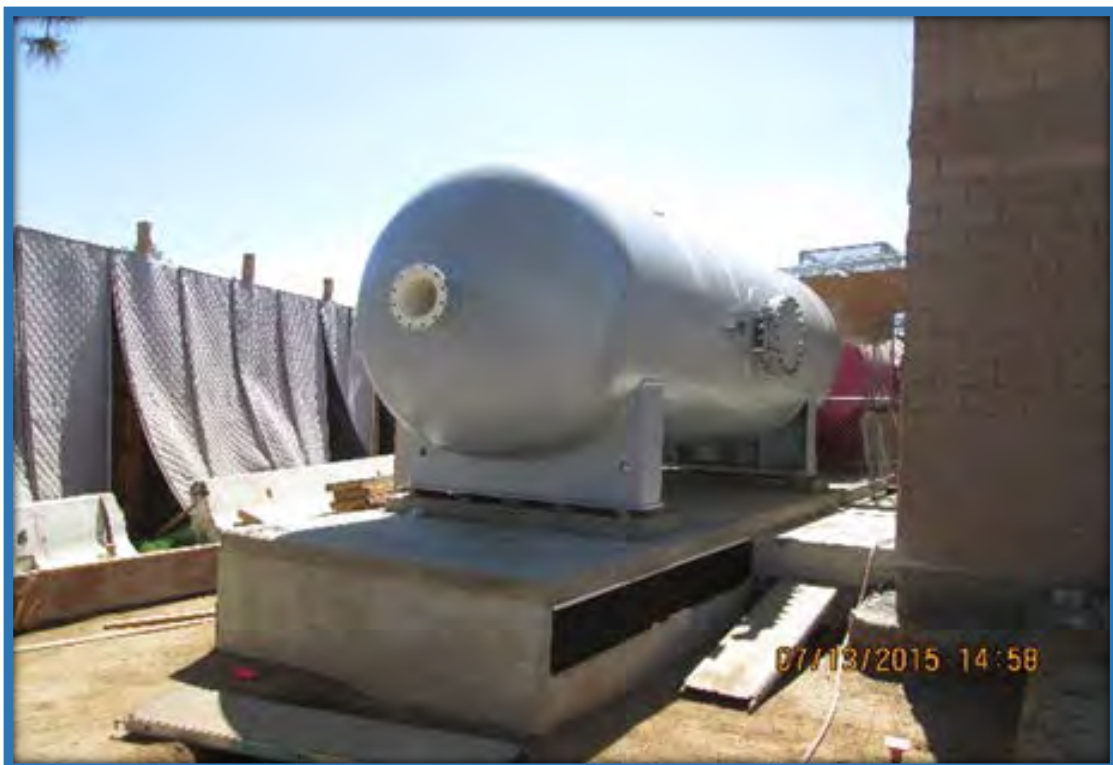
Surge Tank Installed on Pad
