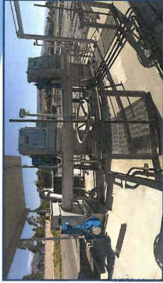
San Luis Obispo Water Resource Recovery Facility Headworks Screening System
