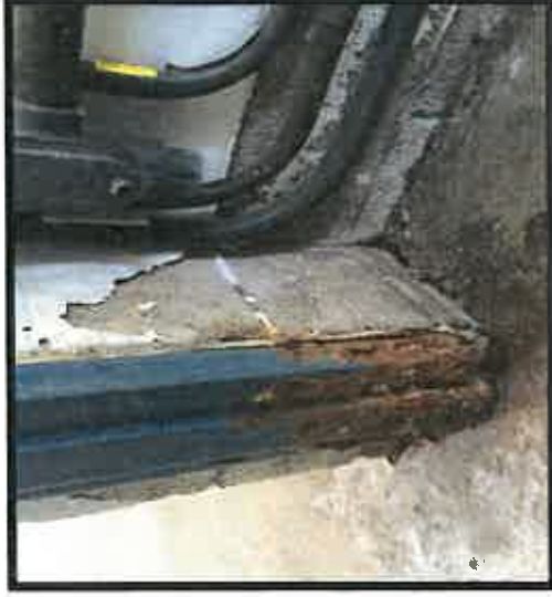
Corrosion from bleach leakage
