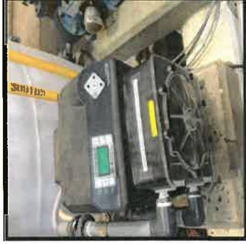
Existing Diaphragm Pump
