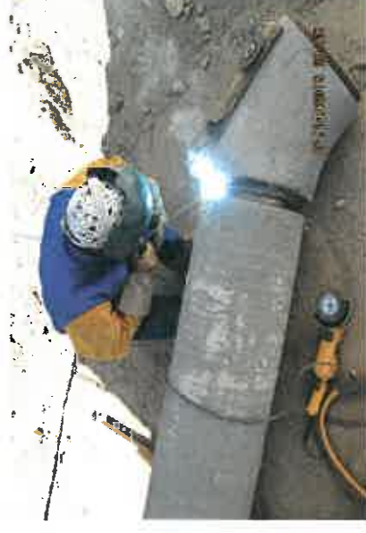
Welding 12-in RW Pipe
