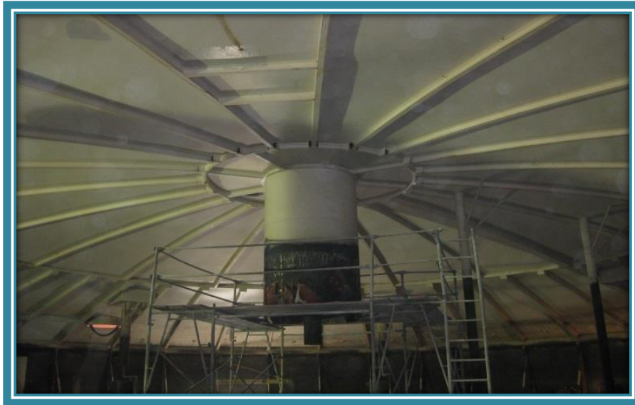
REGIONAL WATER RECYCLING FACILITY NO. 2 – DIGESTER NO. 4 DOME IMPROVEMENTS
