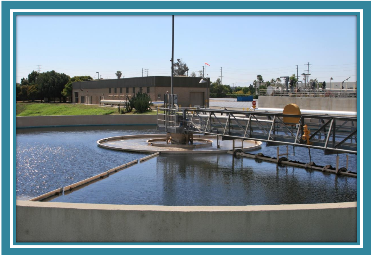
CARBON CANYON WATER RECLAMATION FACILITY
