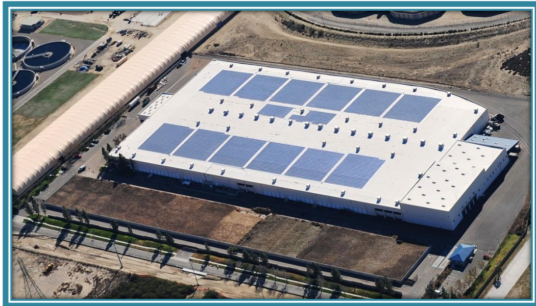
IERCA OVERHEAD VIEW OF SOLAR PANELS
