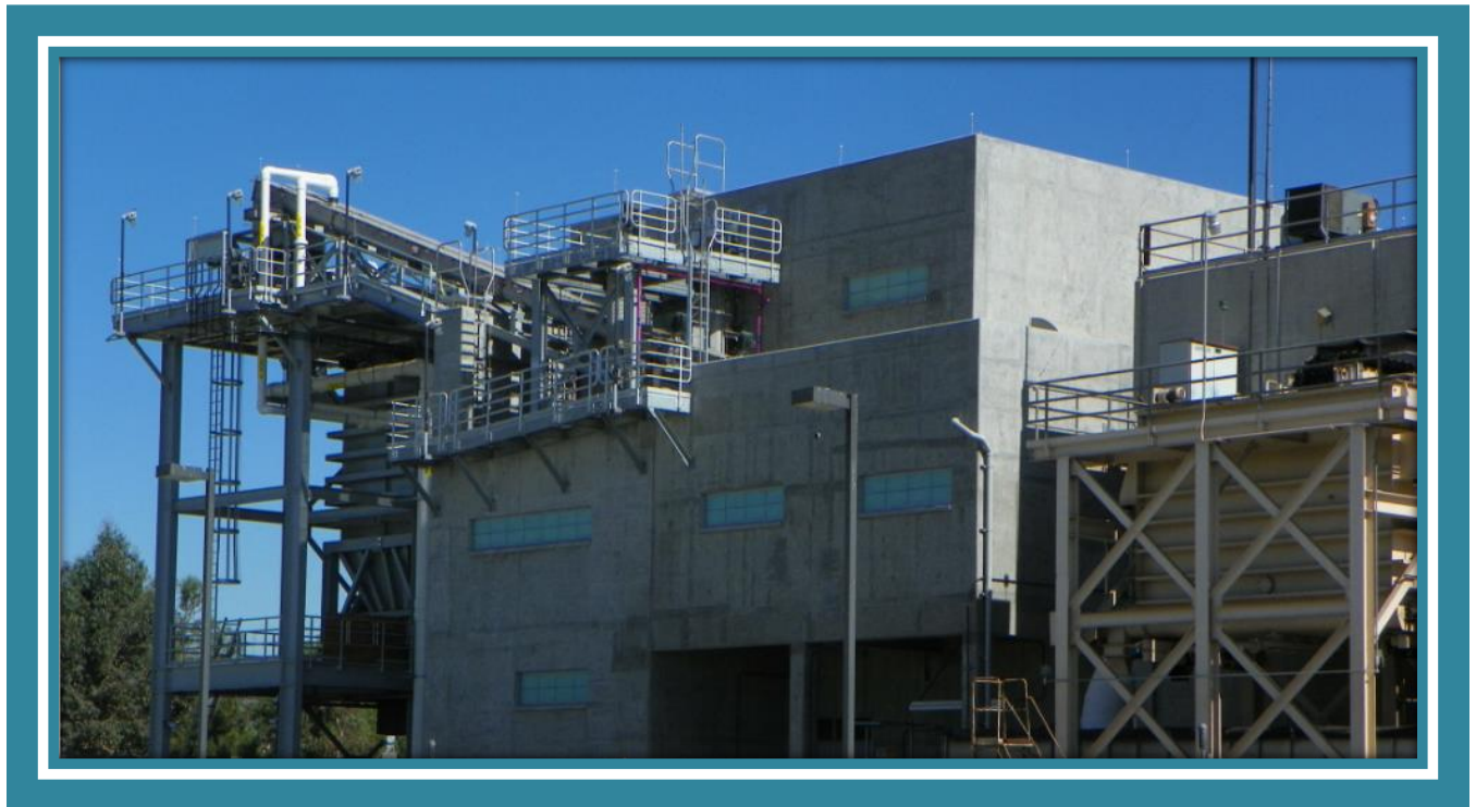
REGIONAL RECYCLING FACILITY NO. 1 DEWATERING BUILDING
