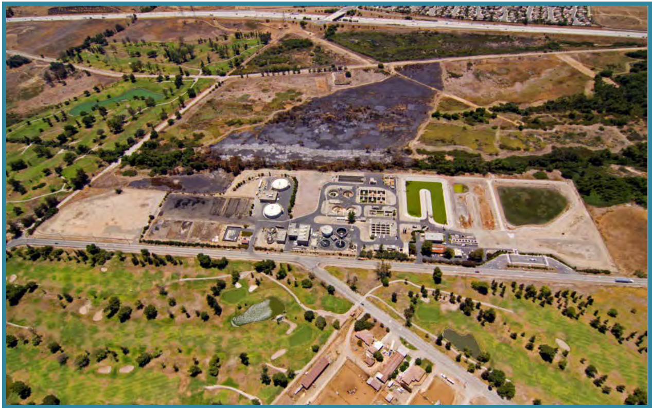
Regional Plant No. 2 (RP-2)
