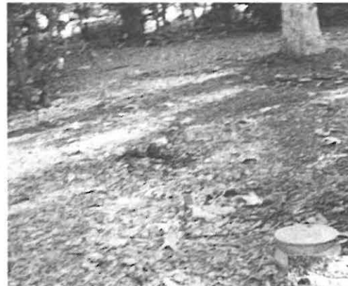
HQ-B Backflow Device - Before
