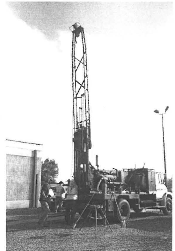
Geotechnical Boring
