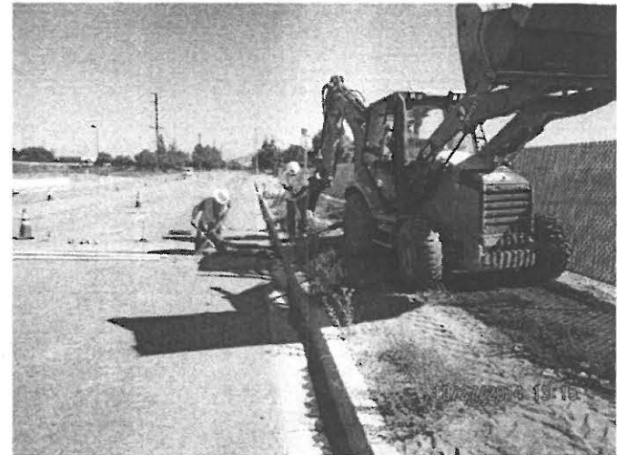
Contractor Mobilization: Electrical Power to Yard
