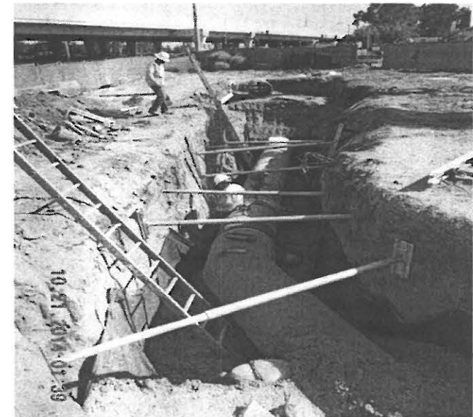
Jack and Bore Pit - Pipe Connection at Eucalyptus and Pipeline
