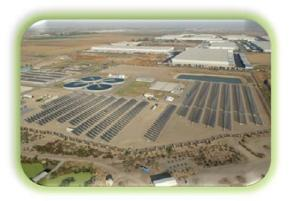
The installation at these sites includes different technologies: roof and ground mounted fixed-tilted panels, horizontal trackers, and tilted trackers. Tilted single-axis tilted tracker, installed at RP-5 just behind IEUA's headquarters, and pictured here, generate 30% more energy than fixed-tilt technology.
