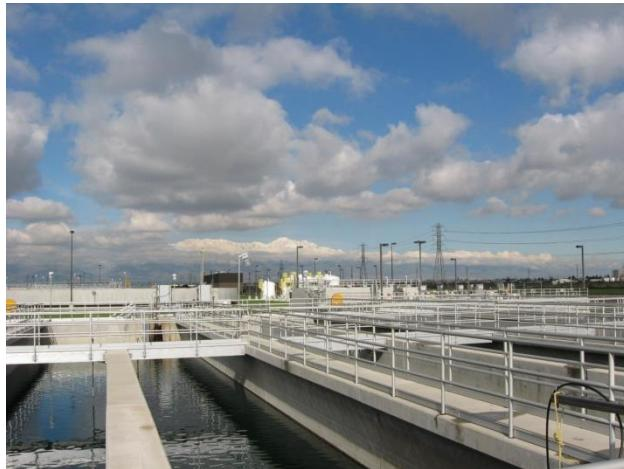
Regional Water Recycling Plant No. 5 (RP-5), located in the City of Chino, has been in operation since March 2004. RP-5 serves the areas of Chino, Chino Hills, Montclair, Ontario, and Upland. Liquids are treated at RP-5, while the solids removed from the waste flow are treated at RP-2. RP-5 treats an annual average flow of 12 MGD.
