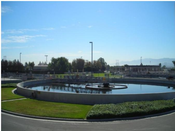
Carbon Canyon Water Recycling Facility (CCWRF), located in the City of Chino, has been in operation since May 1992. The \$46-million facility works in tandem with Regional Plant No. 2 (RP-2) and serves the areas of Chino, Chino Hills, Montclair and Upland. Liquids are treated at CCWRF, while the solids removed from the waste flow are treated at RP-2. CCWRF treats an annual average flow of 9.5 MGD.
