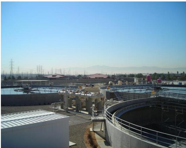
Located in the City of Rancho Cucamonga, the Regional Water Recycling Plant No. 4 (RP-4) has been in operation and producing recycled water since 1997. RP-4 treats an average flow of 11 million gallons per day and is operated in conjunction with RP-1 to provide recycled water to users. The RP-4 facility was recently expanded from its capacity of 7 MGD to 14 MGD. This facility serves portions of Rancho Cucamonga, Fontana and unincorporated areas of San Bernardino County.
