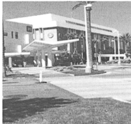
Existing Hospital Building
