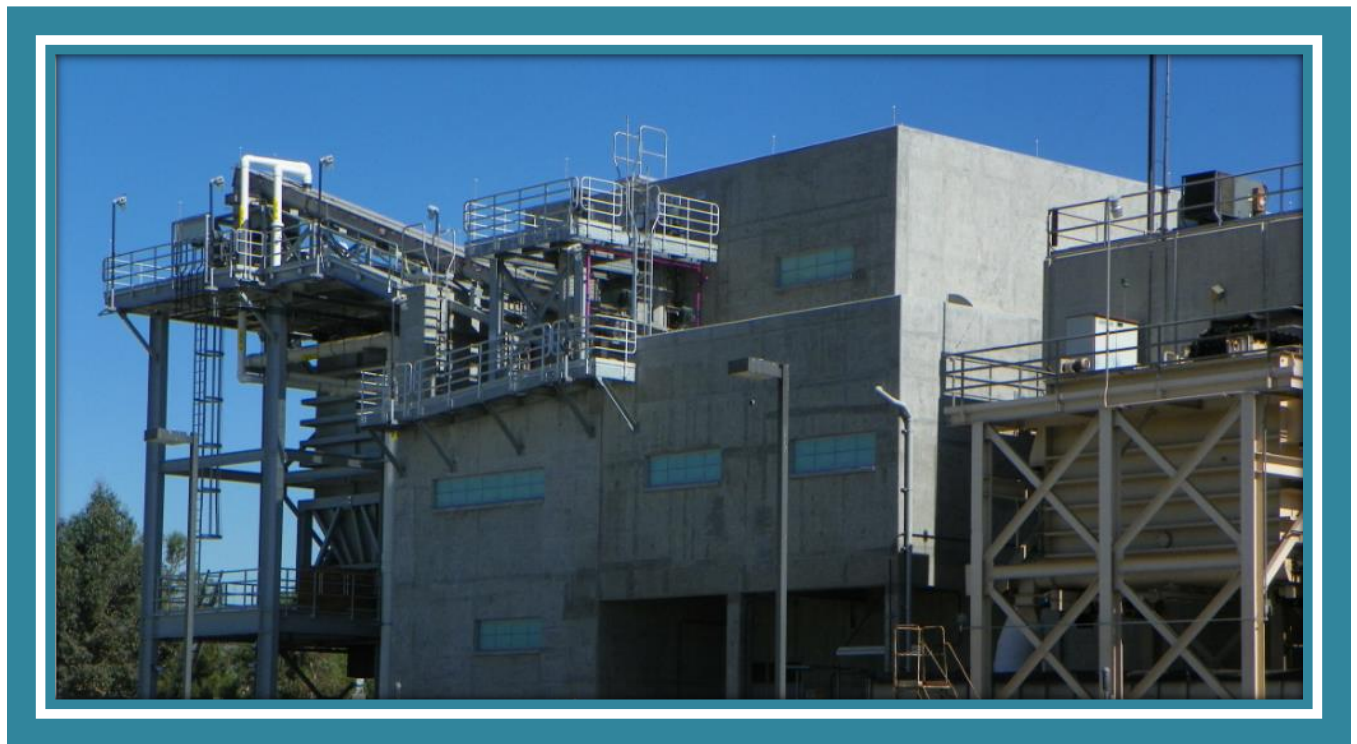
REGIONAL RECYCLING FACILITY NO. 1 DEWATERING BUILDING
