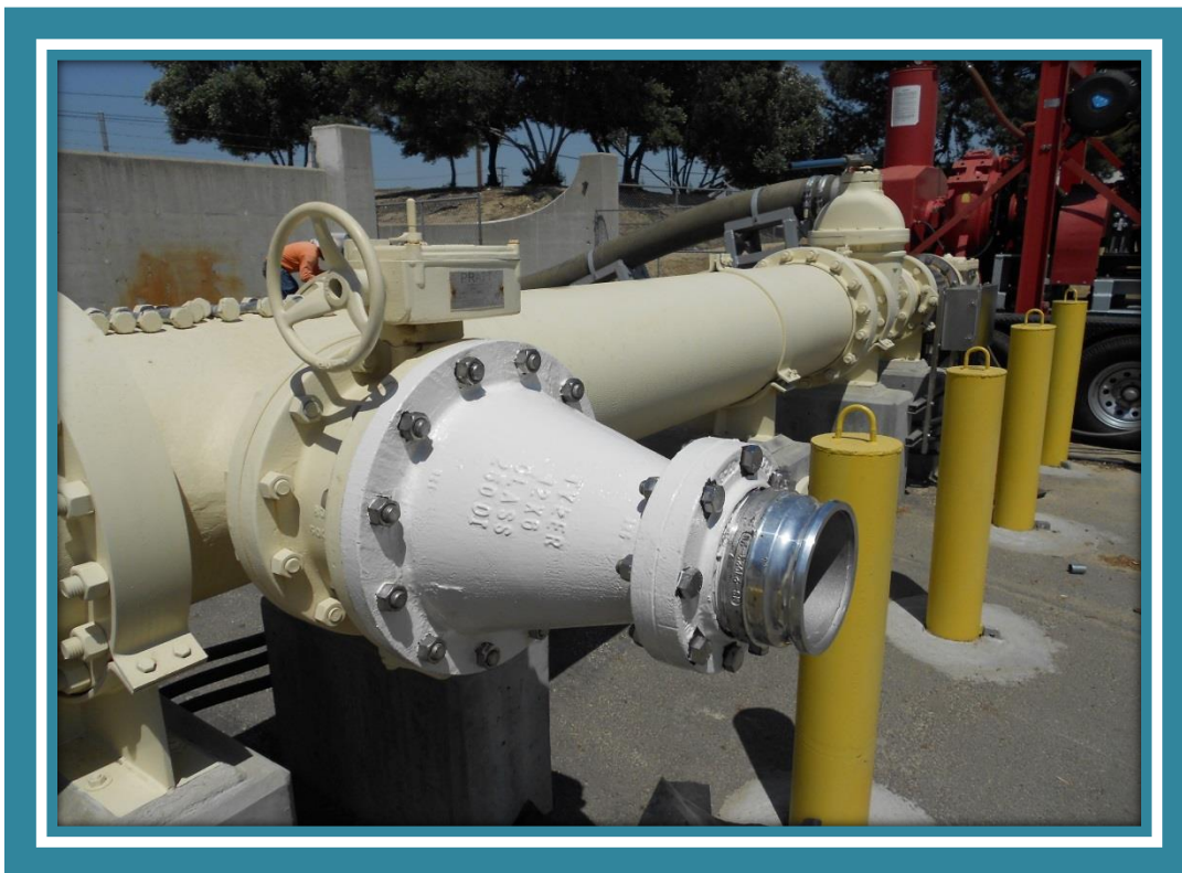
PHILADELPHIA PUMP STATION EMERGENCY BYPASS SYSTEM
