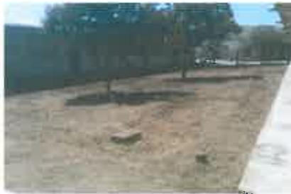
A lot has been going on underground. Irrigation boxes hint to the work that was completed.
