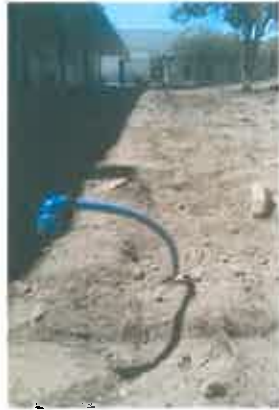
Underground Irrigation is IN! Next on the list are vegetable beds.
