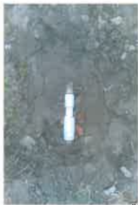
Slip fix used to repair some pipes at Redeemer
