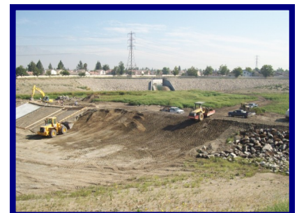
Construction of Berm No. 1 at Declez
