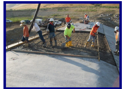
Construction Concrete Spillway at Declez
