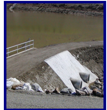
Berm Hardening at Declez Basin
