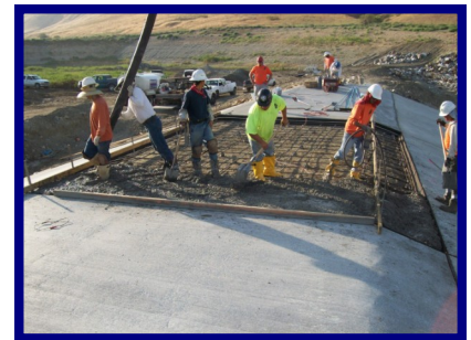
Construction Concrete Spillway at Declez
