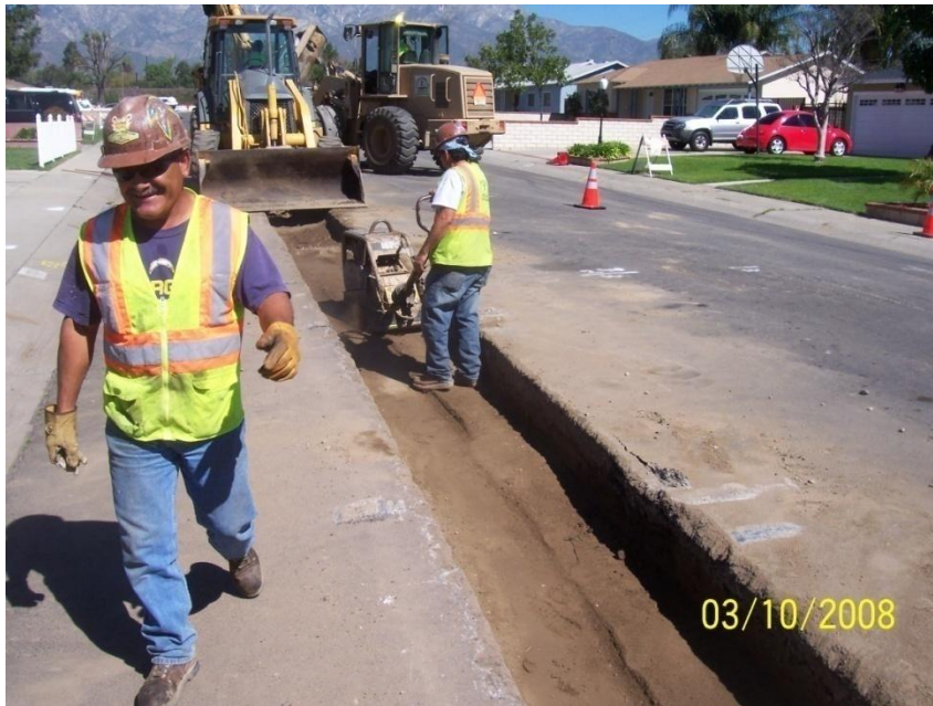
Trench Backfill and Re-compaction on North Council Ave.
