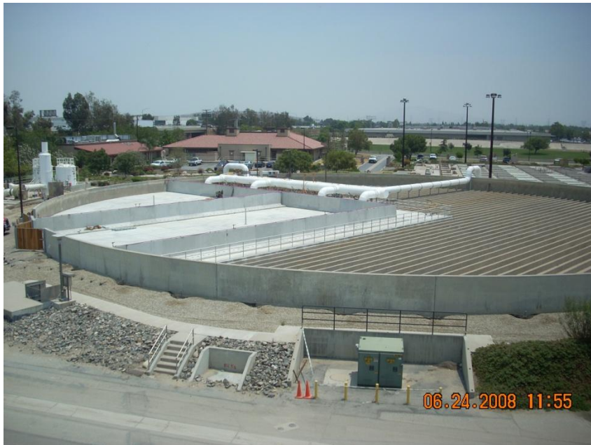
Bio-Filter Structure
