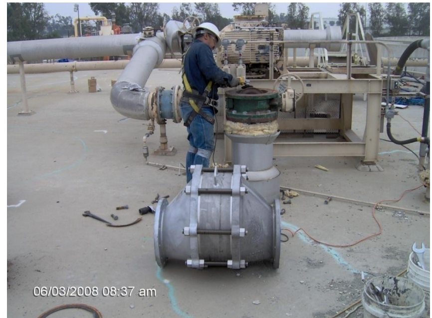
Flame Trap Replacement at Digester #5
