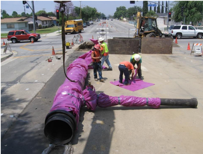
Prepping for installation of 24" RW line with 8" tee and lateral at Orchard St x Monte Vista Ave
