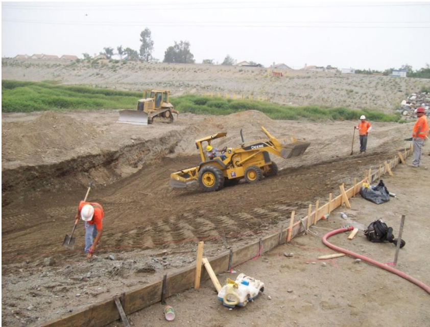
Setting forms for the concrete spillway on Berm no. 1 at Declez Basin
