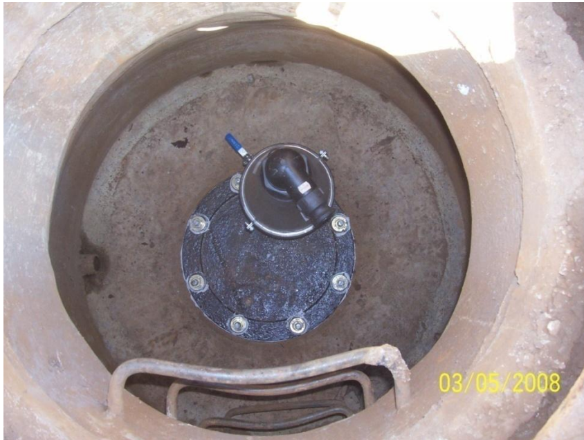
New Pressure lid and air vac on Edison Line City of Montclair
