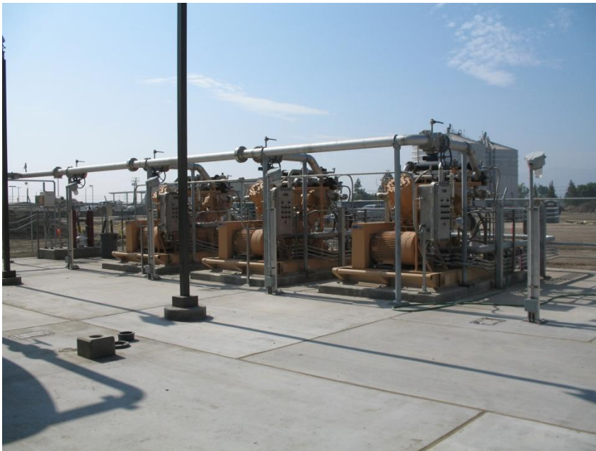
Gas Storage Compressors
