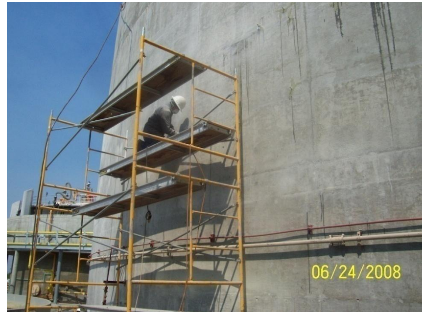
Digester No. 7 Crack Repair
