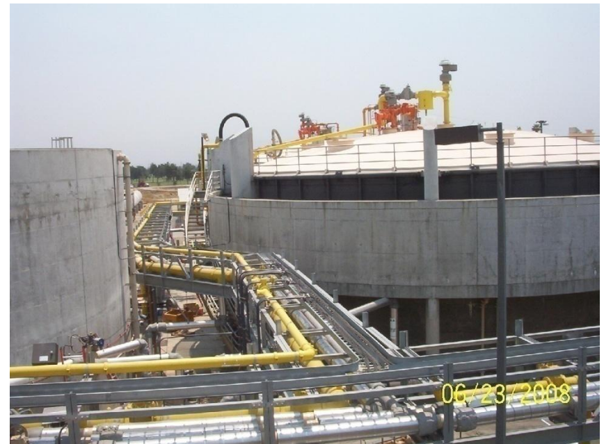
Three Phase Digestion (Pipe Rack #2)
