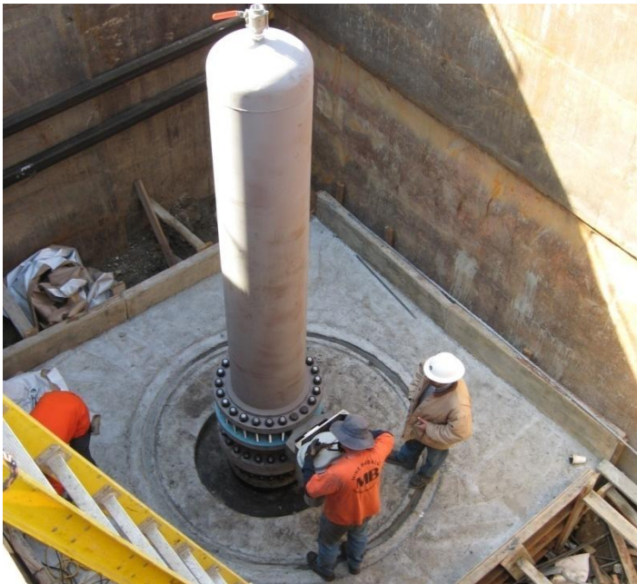
Valve assembly CB20 located in Upland
