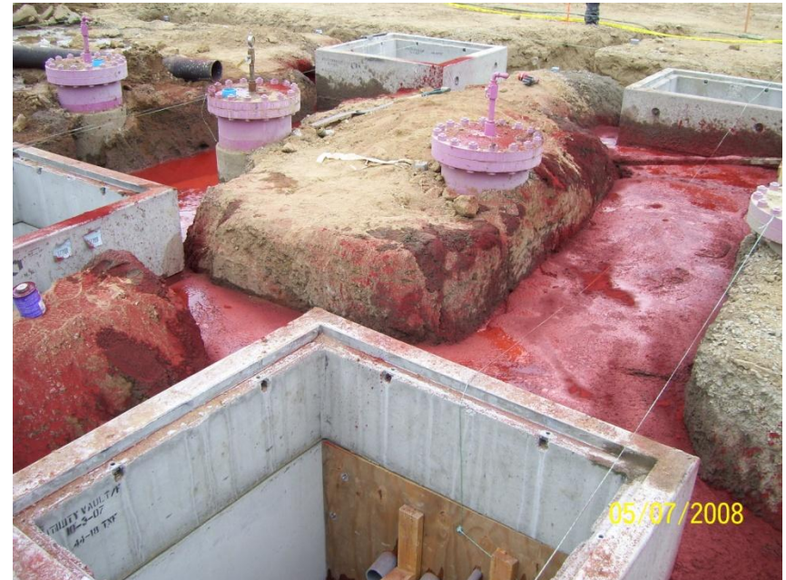
Electrical Duct Banks
