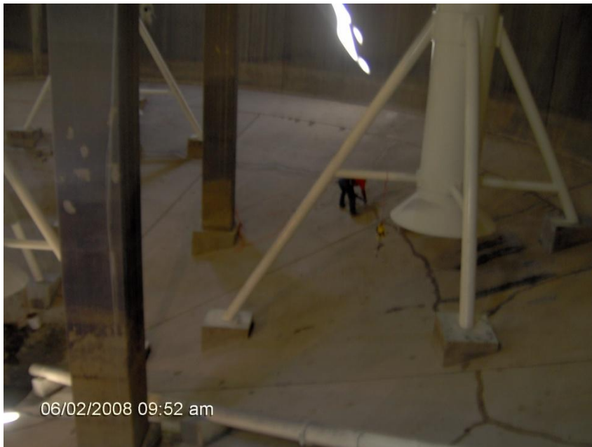
Digester No. 7 Crack Repair Inside Digester
