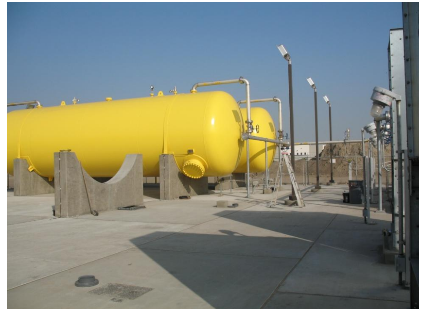
Gas Storage High Pressure Vessels
