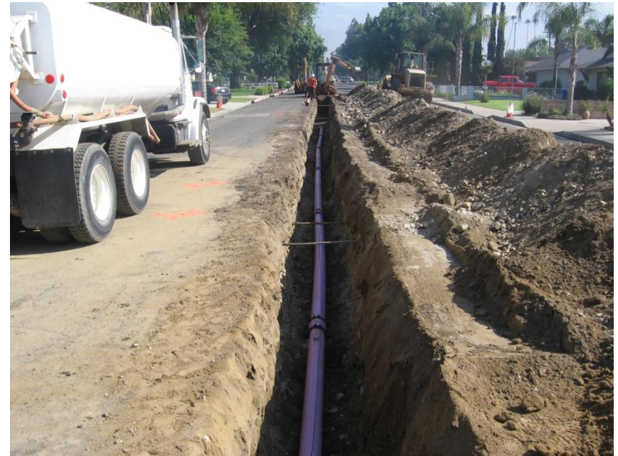
Installation of the 6in MVWD lateral
