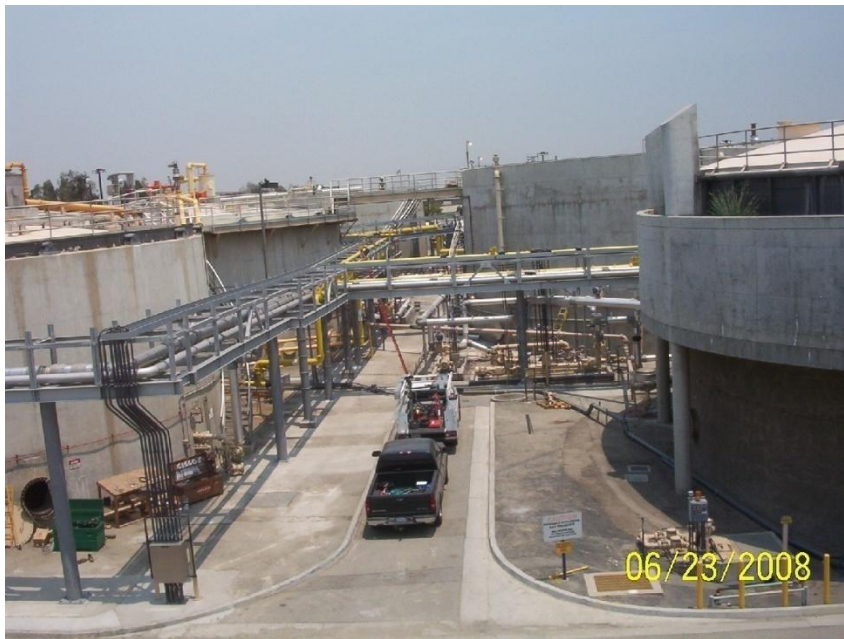
Three Phase Digestion (Pipe Rack #1)
