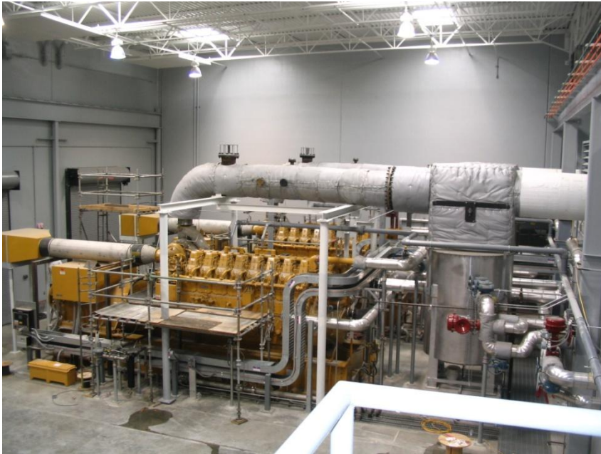
REEP Generators and Heat Recovery Units
