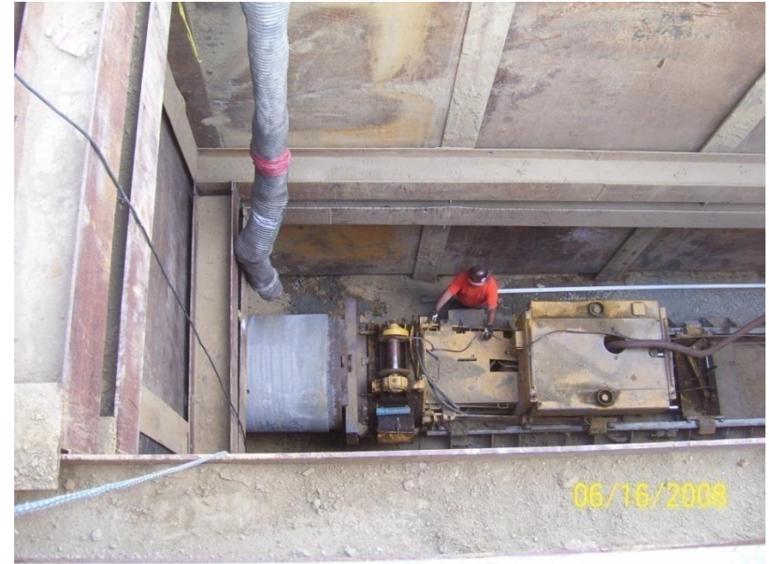
42" CMLC Recycled Water Pipeline Jack and Bore Under MWD 176" raw Water distribution Line
