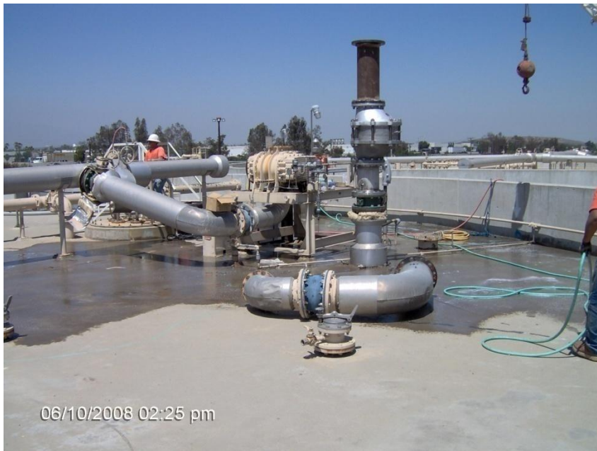
Flame Trap Removal at Digester #5
