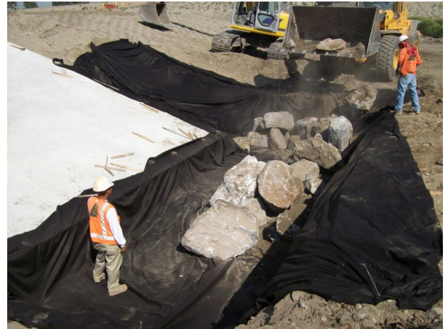
Installing rip rap at toe of spillway of Berm No. 1 at Declez Basin
