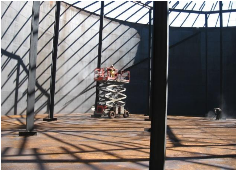
Reservoir# 2 Media Blasting for removal of oils and scale from tank walls
