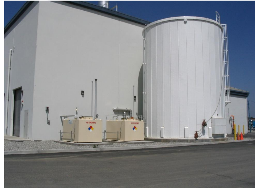
REEP TES Tank and Lube Oil Storage
