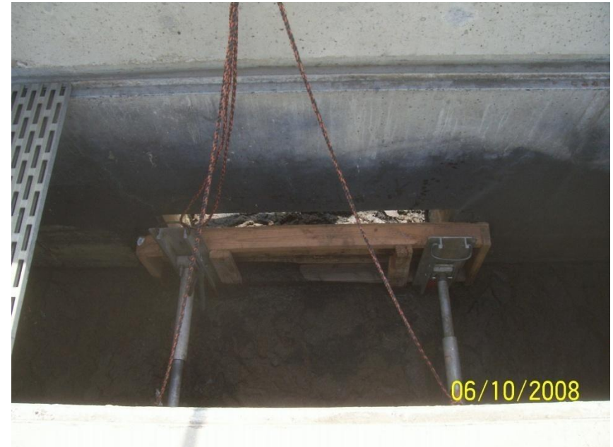
Aeration Basin (Gate Bulk Heading)
