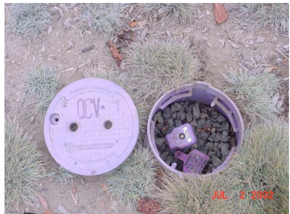
Quick coupler and valve box
