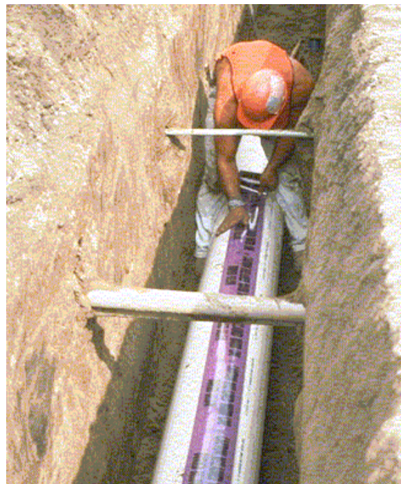
Recycled water pipeline installation with continuous purple warning tape.
