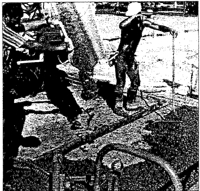
Discharge must be completed within 60 minutes after initial batching or 90 minutes with special admixtures.
