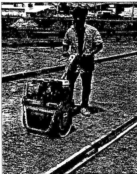
The subgrade is compacted to 92 to 96% of AASHTO T-180, must be moist and free of truck ruts and other irregularities.
