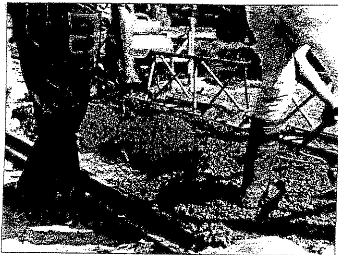
A stiff mix is required with close control of mix water to obtain both permeability and adequate cement-aggregate bond.
