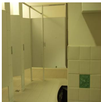
Restroom Partitions and Ceramic Tiles (wall)
