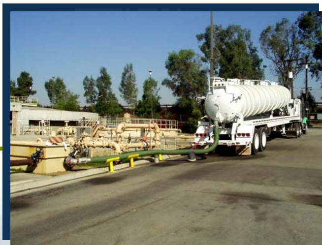
RP-1 Manure Slurry Delivery
