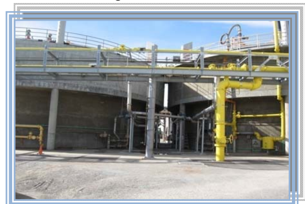
View of the Newly Installed Gas Piping from Digesters No. 1 and No. 2
