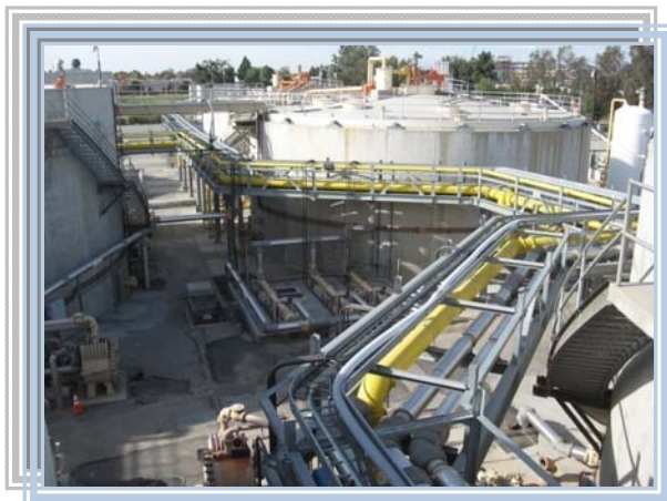
RP1-Newly Installed Overhead Gas Piping
