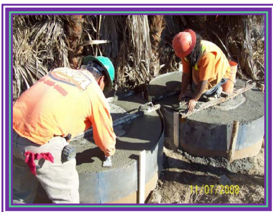
Installation of New Manhole Rings and Covers at the NRW Line
