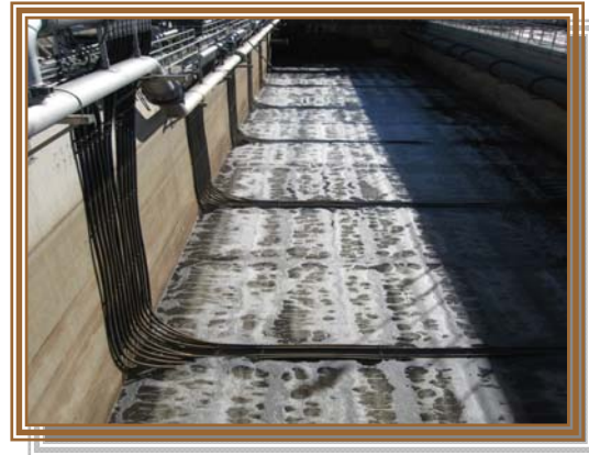
Carbon Canyon - Testing of Aeration Panels
