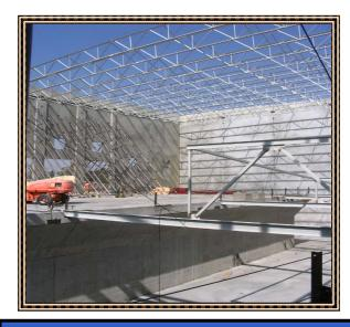
**Steel Trusses for Conveyor Supports**
