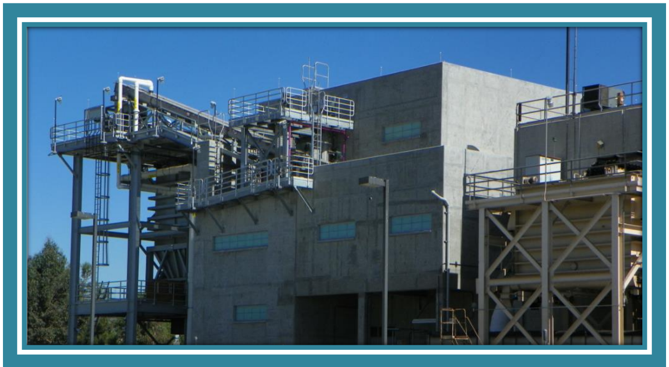
REGIONAL RECYCLING FACILITY NO. 1 DEWATERING BUILDING
