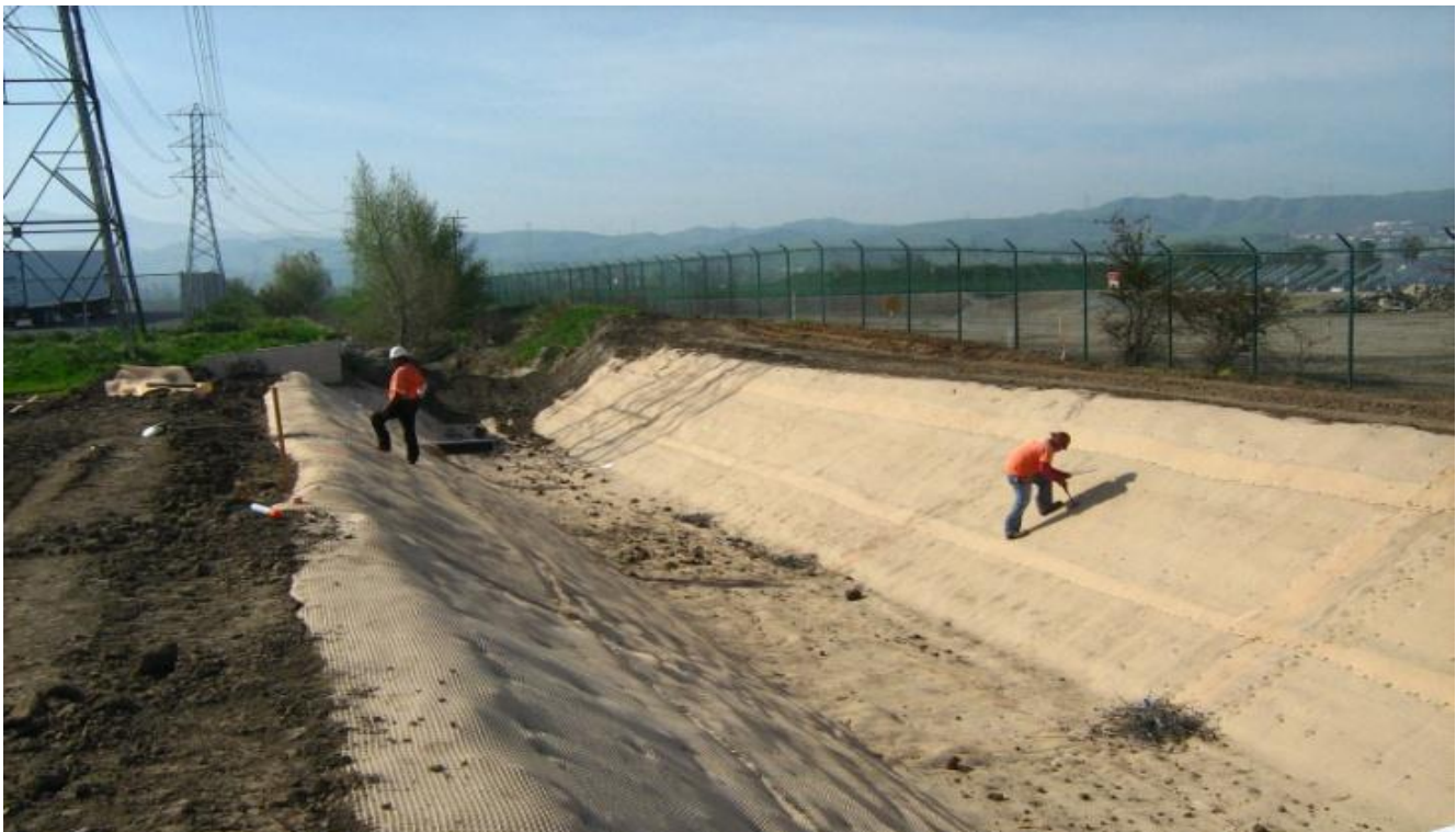
Magnolia Channel Project - Chino, CA
