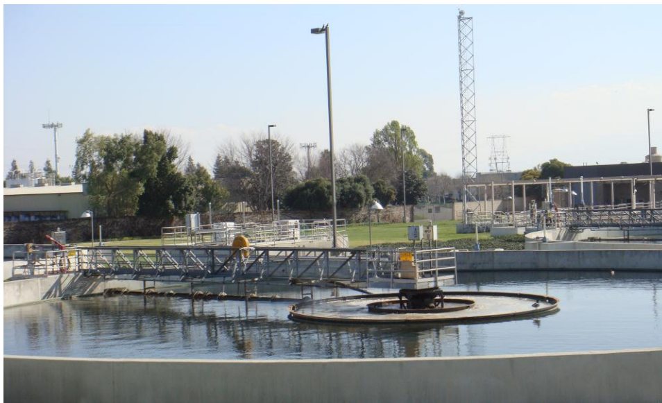
Secondary Clarifier Carbon Canyon Wastewater Reclamation Facility
