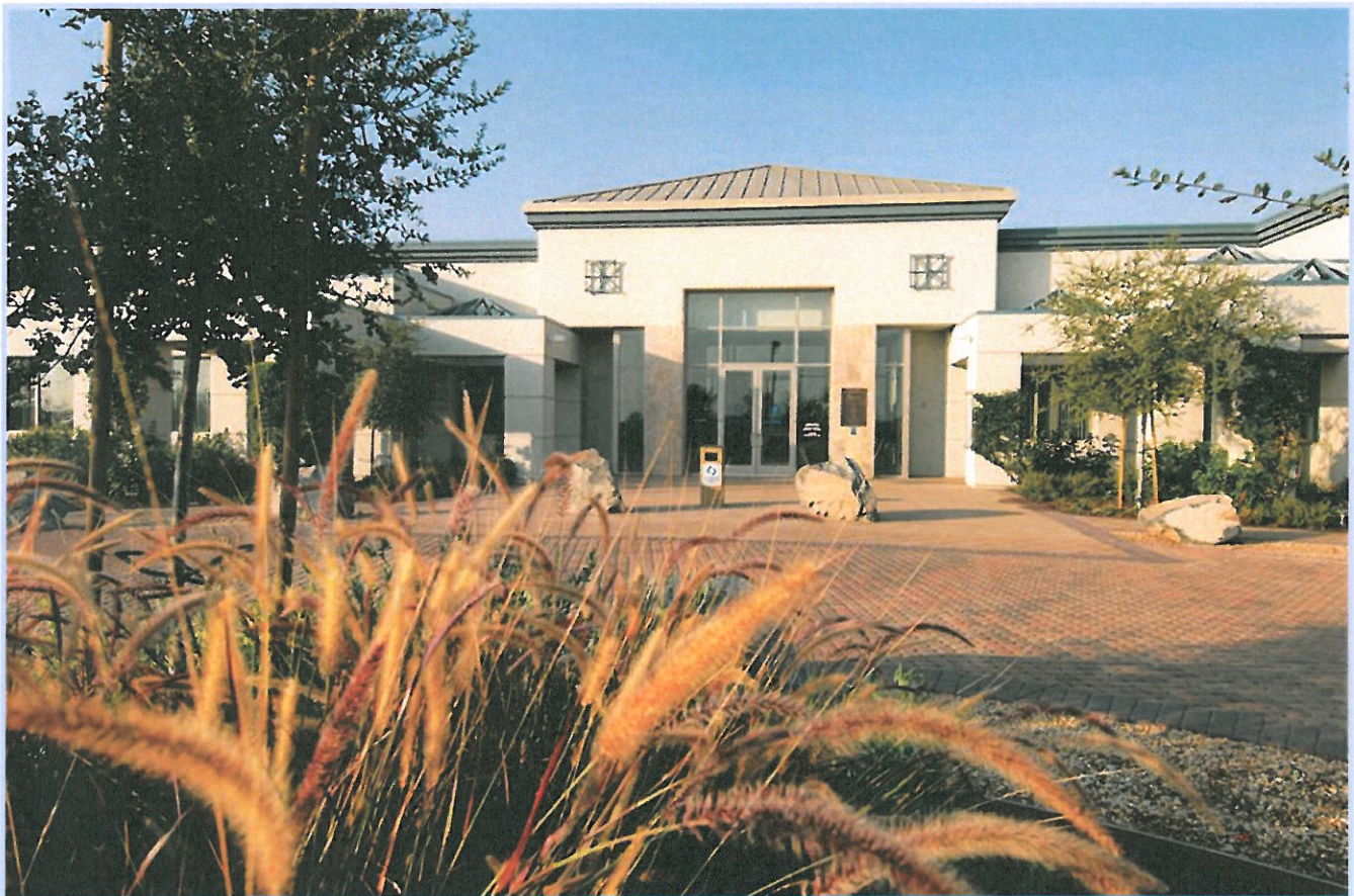
Agency Headquarters Building A in Chino, CA.
