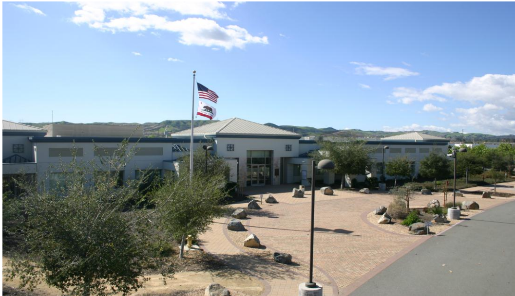
IEUA Headquarters Building in Chino, CA
