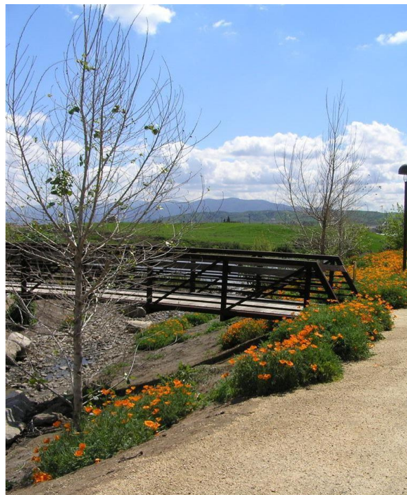
Headquarters Building Bridge
