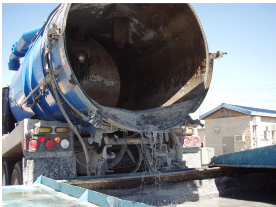
Pipeline Cleaning Discharge- IEUA Vactor Truck
