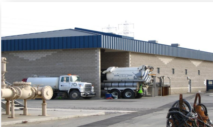
RP-1 Maintenance Facility – Ontario, CA
