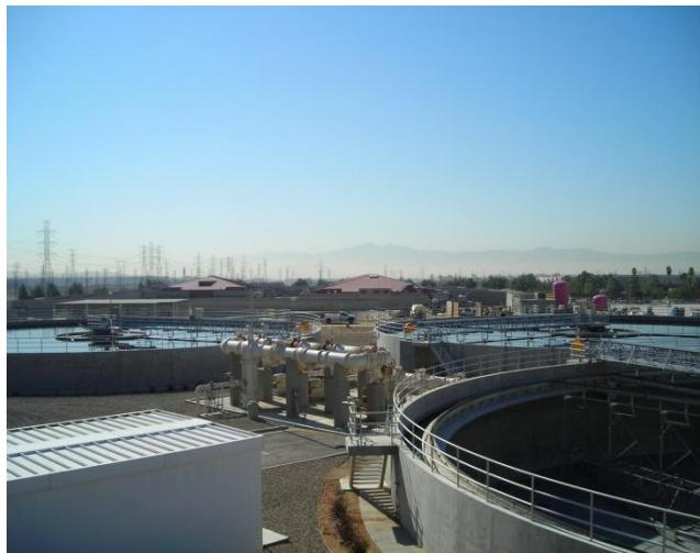
Located in the City of Rancho Cucamonga, the Regional Water Recycling Plant No. 4 (RP-4) has been in operation and producing recycled water since 1997. RP-4 treats an average flow of 5 million gallons per day and is operated in conjunction with RP-1 to provide recycled water to users. The RP-4 facility was recently expanded from its capacity of 7 MGD to 14 MGD. This facility serves portions of Rancho Cucamonga, Fontana and unincorporated areas of San Bernardino County.
