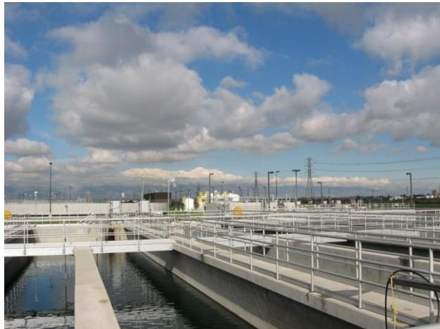
Regional Water Recycling Plant No. 5 (RP-5) is located in the City of Chino, has been in operation since March 2004. RP-5 serves the areas of Chino, Chino Hills, Montclair, Ontario, and Upland. Liquids are treated at RP-5, while the solids removed from the waste flow are treated at RP-2. RP-5 treats an annual average flow of 12 MGD.
