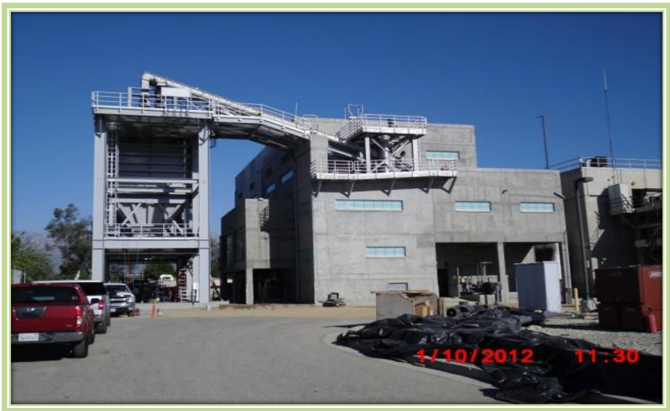
Regional Plant No. 1 – Ontario, CA
