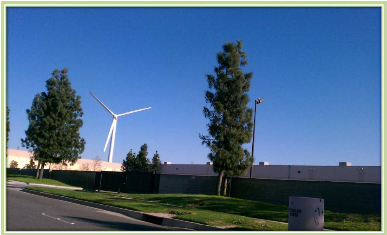
Wind Turbine – Regional Plant No. 4 – Rancho Cucamonga, CA
