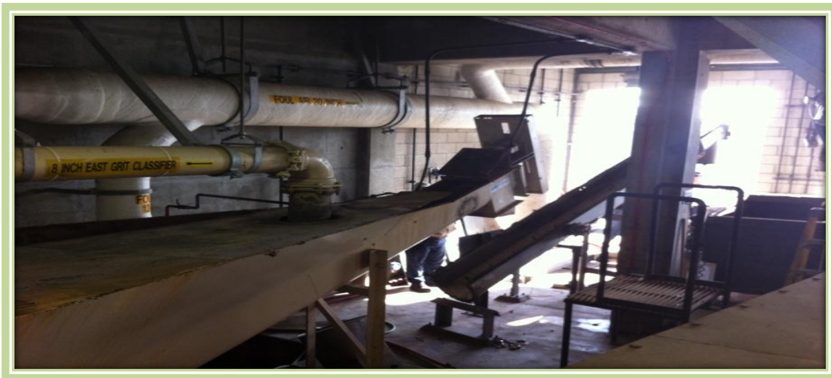
Regional Plant No. 1 – Grit Conveyance Modifications
