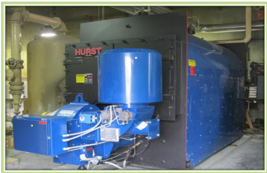
Boiler Replacement Project - Regional Plant No. 1 - Chino
