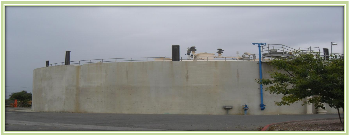
Regional Plant No. 2 Digester No. 3- Chino, CA
