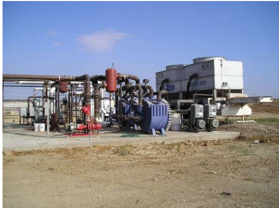
Central Plant (cooling tower and absorption chillers)
