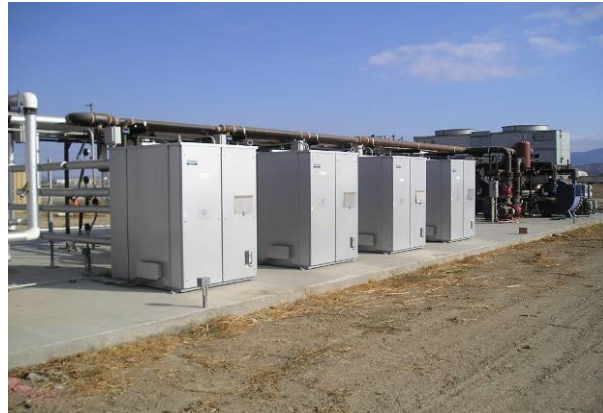
Central Plant (cooling tower and absorption chillers)
