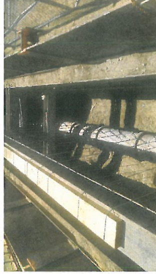
Casing Extension on 27" Regional Sewer on Union Pacific Railroad Crossing
