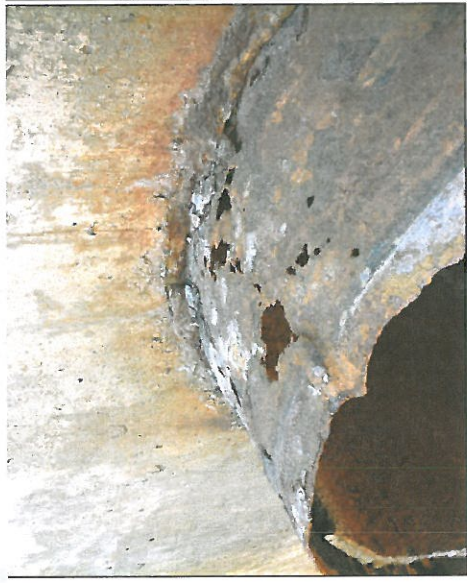
Severe Corrosion
