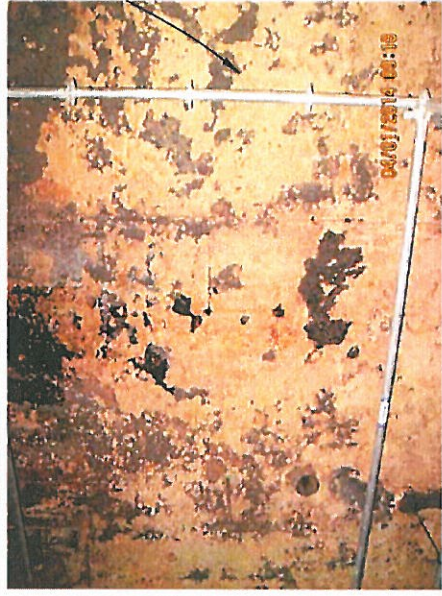
Digester interior wall
