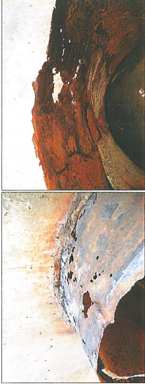
Figure 3 - Severe corrosion of welded steel cylinder at bladder valve vault pipe access point
