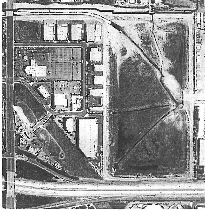
Wineville RWPL Segment B in Day Creek Channel
