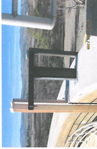
Annular Space between Digester Skirt and Wall
