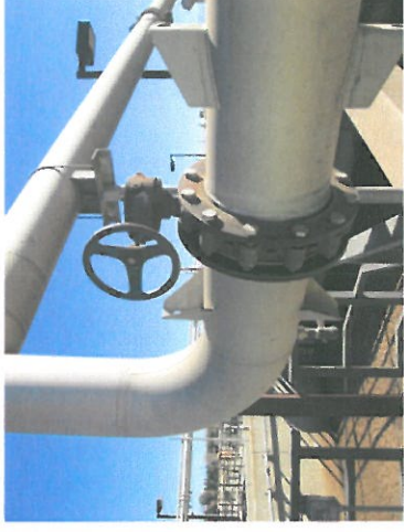
Butterfly Valve Replacement
