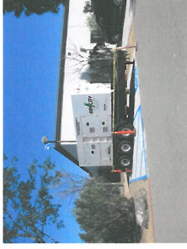
Temporary Generator Supplying Power to HQ During Shutdown
