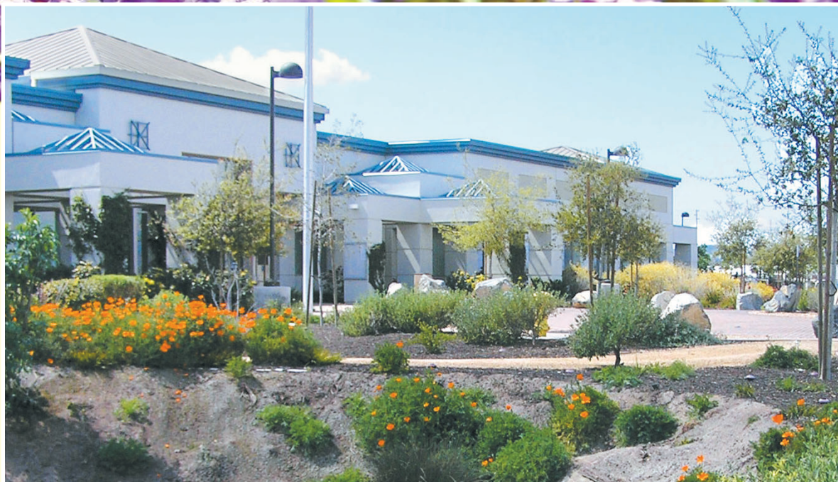
IEUA award-winning, energy-efficient headquarters
