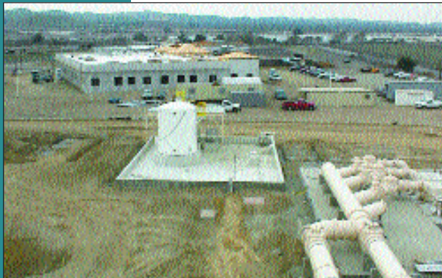
Regional Plant No. 5 and IEUA's New Headquarters, December 2002
