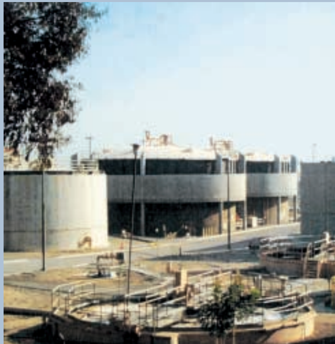
Digesters at Regional Water Recycling Plant No. 1 in Ontario.
